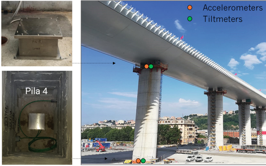
Fig. 5. The position of the fiber optic accelerometers and tiltmeters at the base and head of each pile.
