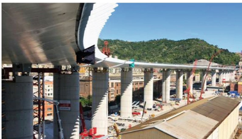
Fig. 2. The Genoa San Giorgio Bridge: a mixed steel-concrete structure with 18 concrete pillars and a 1km long steel deck made of 19 spans.
