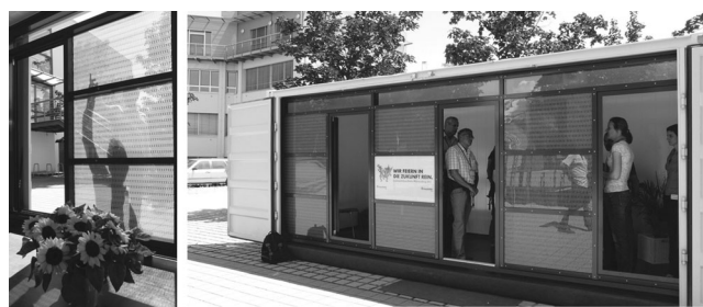
Figure 3. Showroom for BIPV applications of large-area, glass-frit-sealed DSC modules (meander type), as developed at Fraunhofer ISE (2012).
