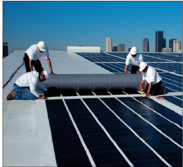
Figure 6. An example of Uni-Soar laminates on a rooftop.
