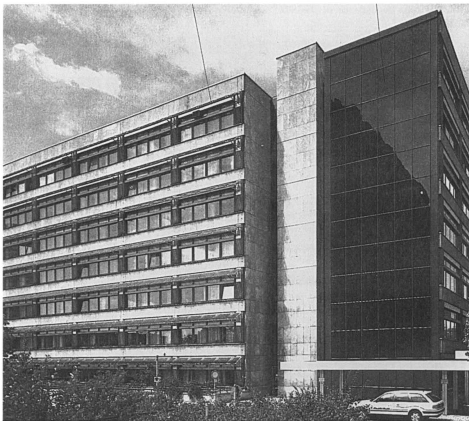
Fig. 9. Photovoltaic facade, Bavarian State Ministry for Environmental Affairs, Munich, Germany: 264 modules of 0.6 \times 0.9 \text{ m}^2 , arranged in 66 panels of 4 modules each, a-Si/a-Si tandem cell structures, 6 kW at 120 V dc.
