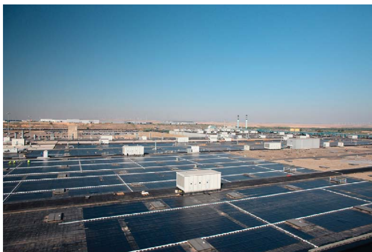
Figure 44 World's largest roof-top PV system (12 MW) in Zaragoza, Spain, deploying a-Si:H PV products.
